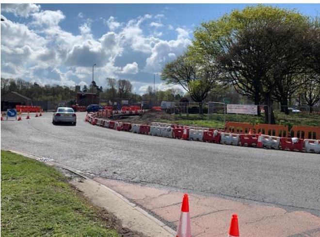
construction works and to improve driver visibility. During the night works, Dyer & Butler excavated and reinstated carriageway crossings on all the approach roads of Farmers Roundabout.
