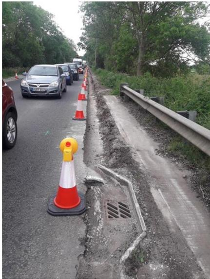
To the North of Farmers Roundabout, we will continue installing new kerb lines and lay the foundation layers within the road widening areas. You may also notice the installation of the new traffic signal furniture and associate control equipment.
