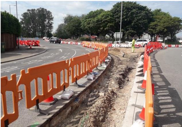
In undertaking the works so far, we have encountered a few problem areas that have been mainly associated with buried underground services such as gas, water, electric mains, and telecommunication cables.
