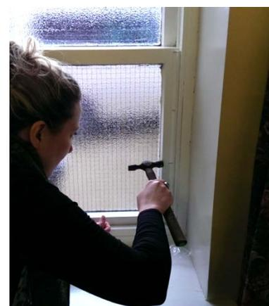
use the bradawl with firm pressure to make a hole about 10mm from each end of the strip.
