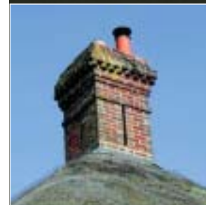
fig 85. Chimney with corbelled brickwork
