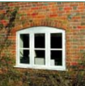
fig 82. Arched brick lintel, small panes
