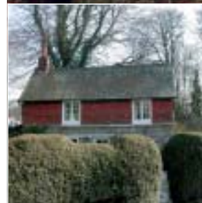
fig 46. Decorative hung tiles Slate roof
