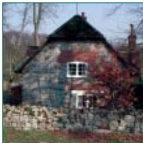
fig 44. Sarsen, flint and brick walls Low Sarsen boundary walls Semi-hipped roof (7)
