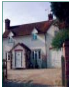
fig 59. House built c1950, extension on right
