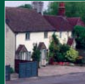
fig 98. Cottages on the Main Road
