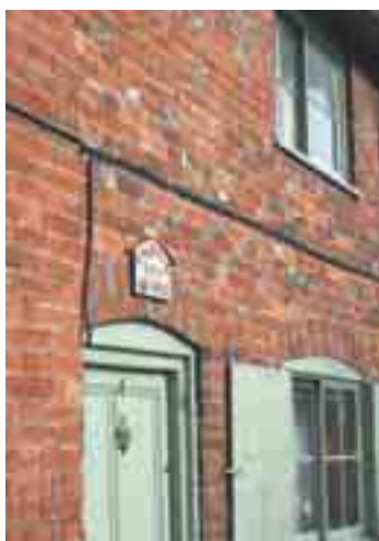
Sliding sash window over upper storey with brick flat arch over
