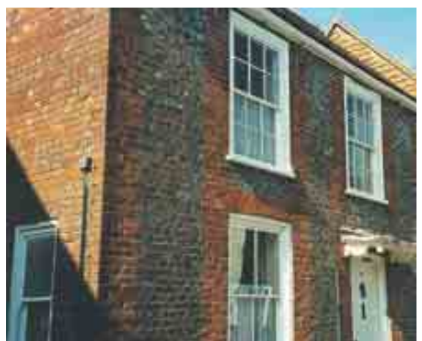
Sash windows and typical door hood
