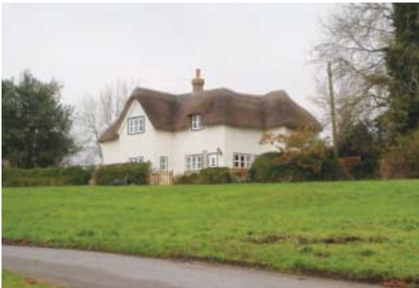
Upper Chute, Village Green
