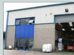
Photos: SIMS recycling state of the art WEEE recycling facility in Mississauga, Ontario, Canada (image courtesy of SIMS Recycling Solutions) WEEE recycling facility, Mallusk, Northern Ireland (image courtesy of AMI)
