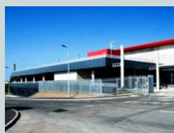
Photos: WTS, Bangor (image courtesy of Heron Bros. Ltd)
