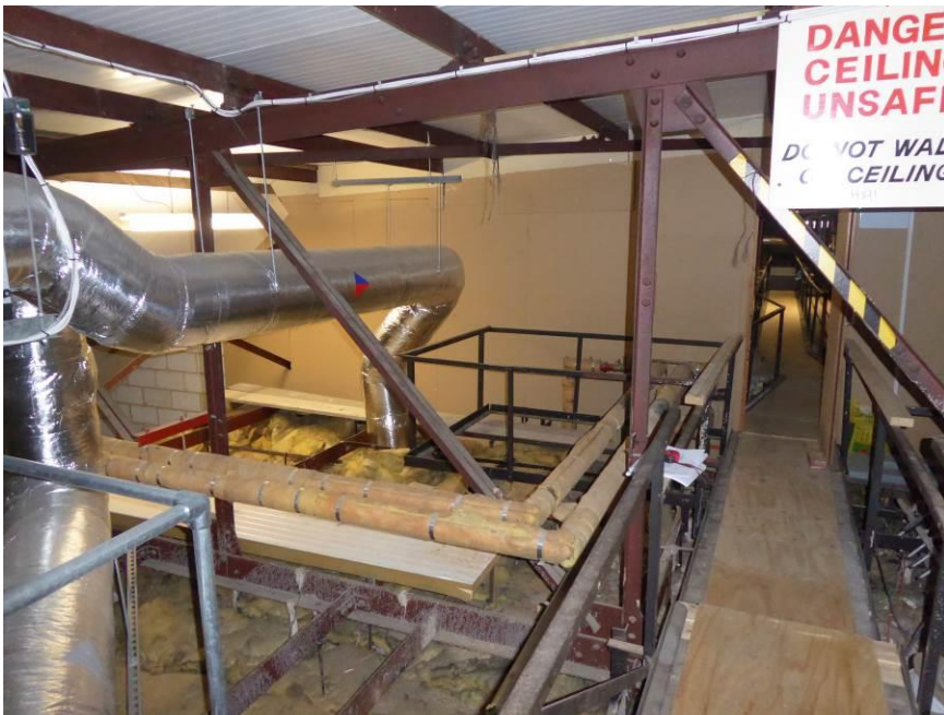
Photograph A18 – loft over Alemein Room.
