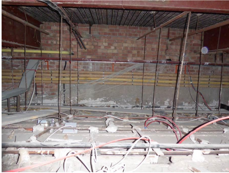
Photo 2 – ceiling void above Foyer.
