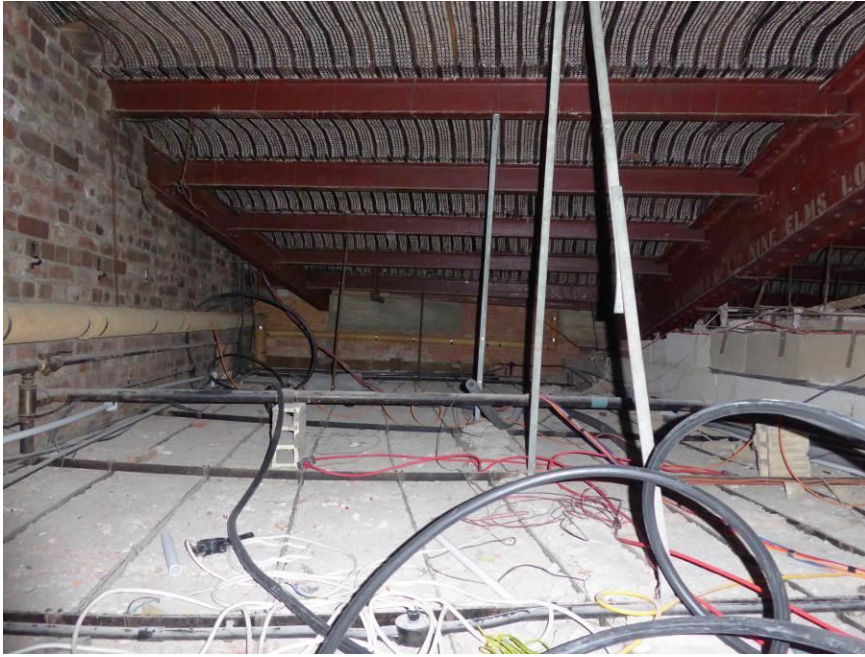
Photograph A13 – ceiling void over Kitchen / Servery.
