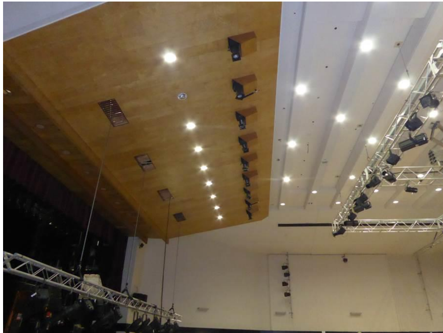
Photo 22 – lighting platform, underside view.
