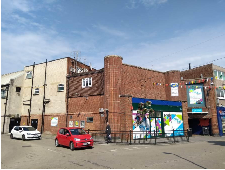
Photograph A7 – Front / South elevation.
