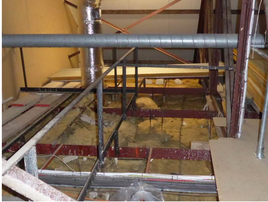
Photo 27 – ceiling above Almein Room.
