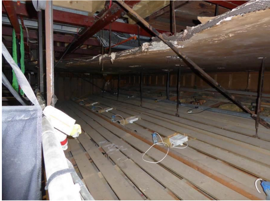
Photo 21 – suspension of the lighting platform.
