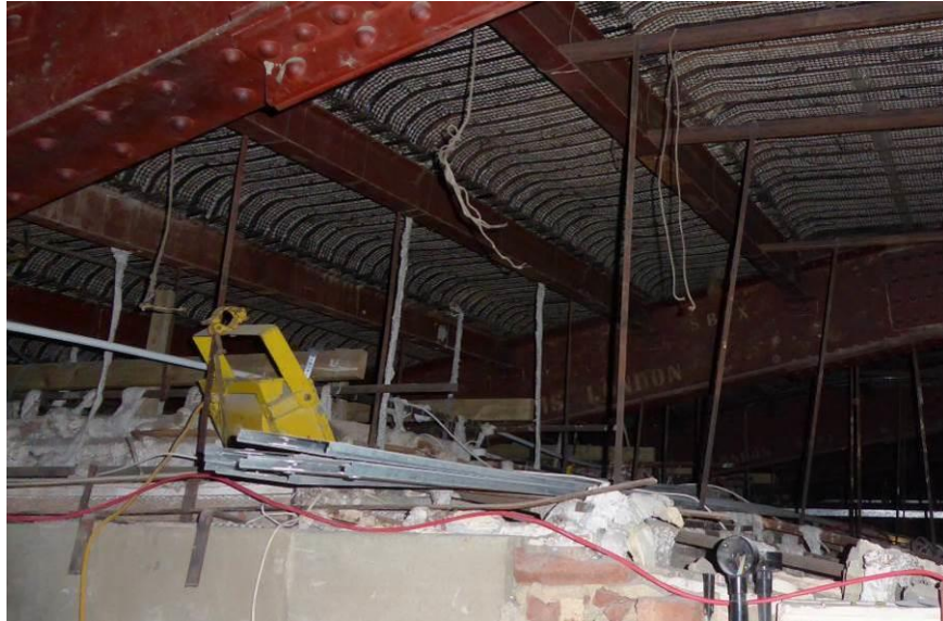
Photo 6 – void over Foyer ceiling, timber frames over the coffers.
