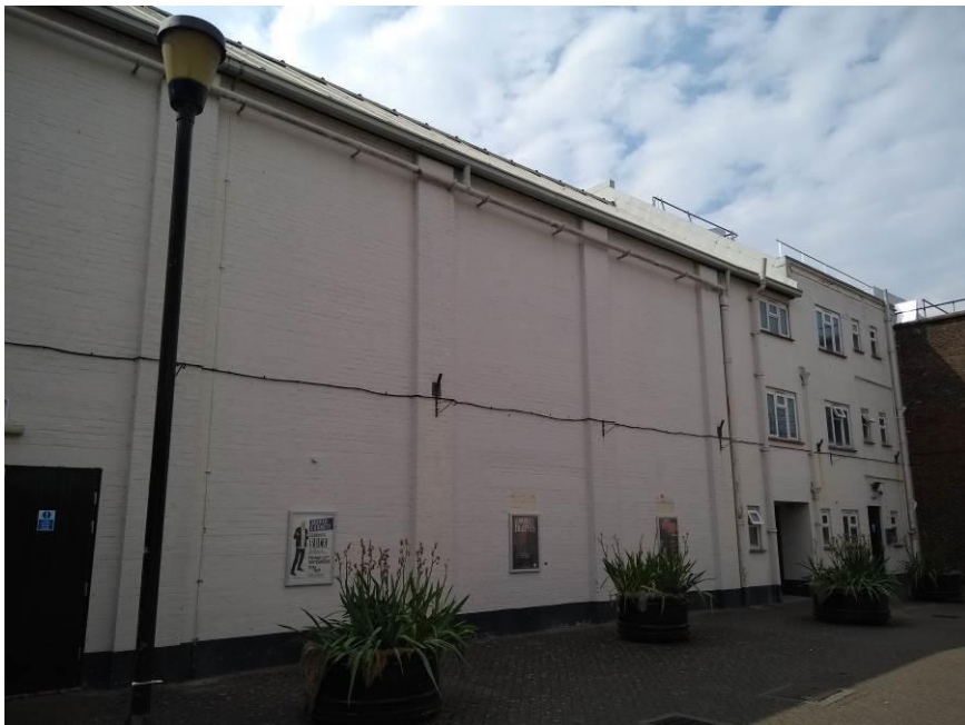
Photograph A2– East / side elevation, auditorium external wall.
