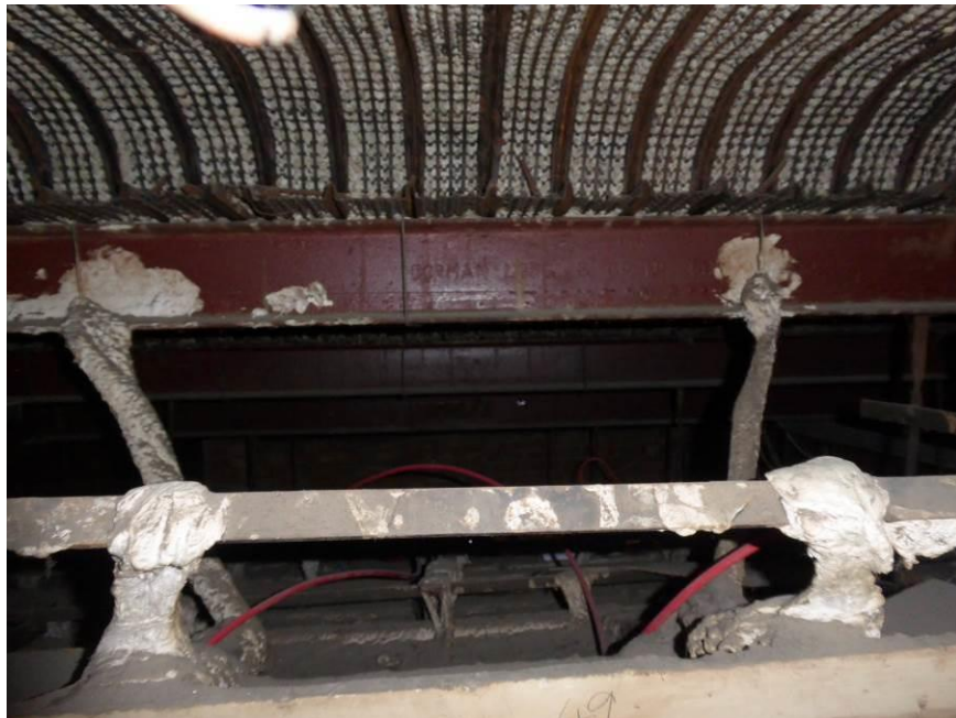
Photo 3 – hessian wadding ties supporting the suspended ceiling.
