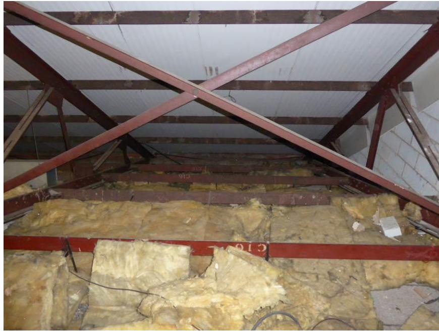
Photo 18 – void over vaulted ceiling.
