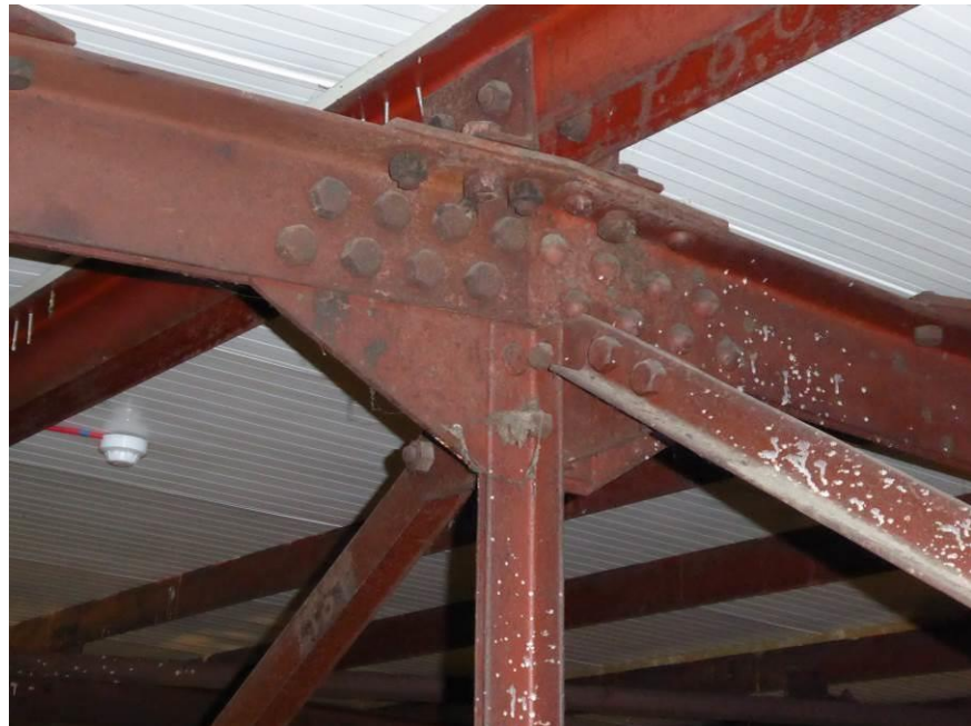
Photo 12 – truss connection.
