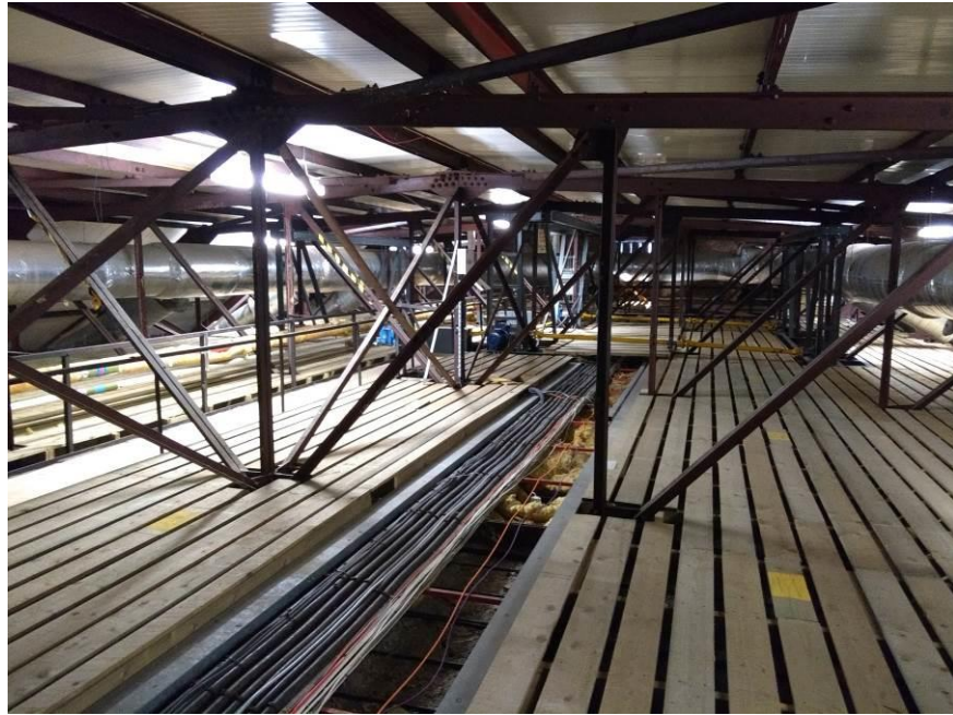
Photo 11 – loft above Auditorium.
