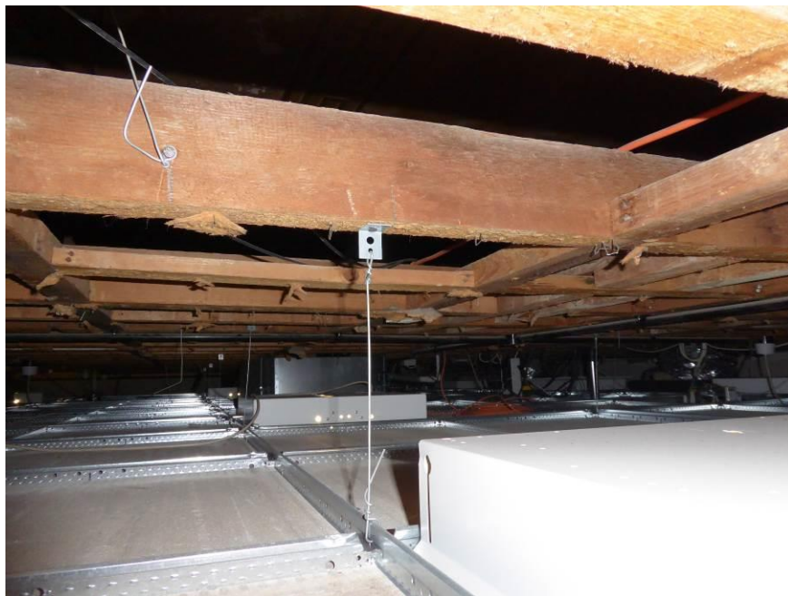
Photo 31 – Tiled suspended ceiling and timber frame over Alemein Room.
