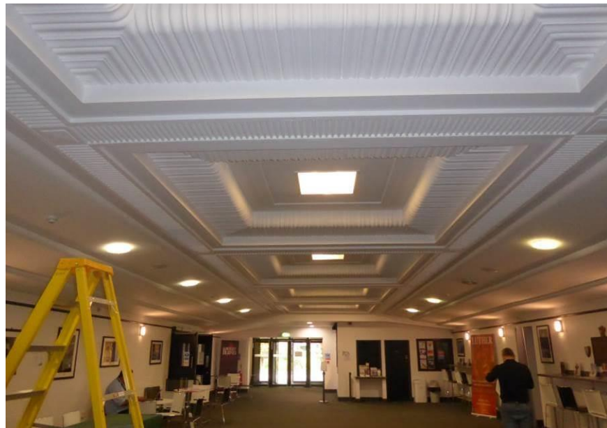
Photo 4 – The suspended ceiling over Foyer.
