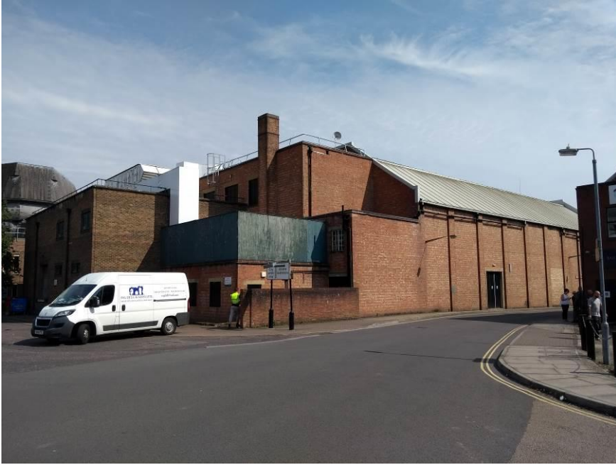
Photograph A5 – West elevation, North end.
