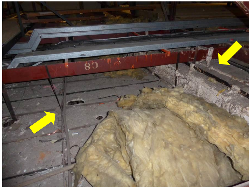
Photo 17 – suspended ceiling, visible junction with high level ceiling.
