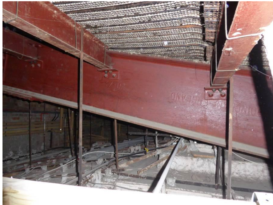
Photo 1 – ceiling void above Foyer.
