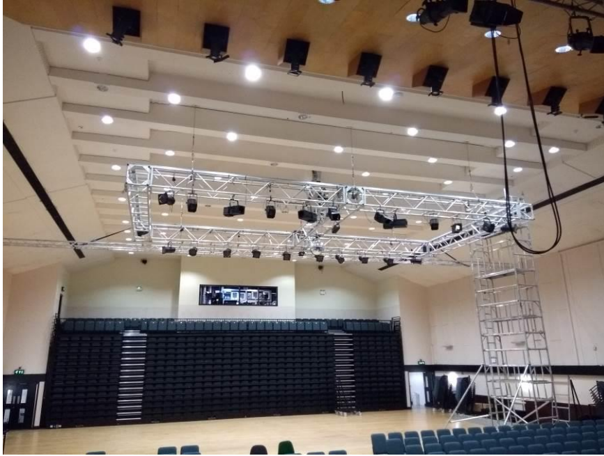
Photograph A11 – auditorium, view towards rear wall.
