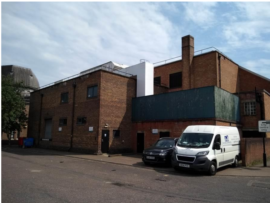
Photograph A4 – North elevation.
