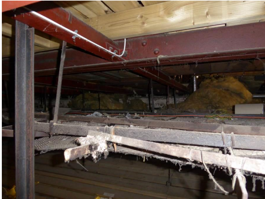
Photo 19 – historic ceiling substructure.
