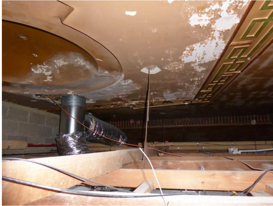
Photo 30 – The underside of suspended ceiling over Alemein Room.
