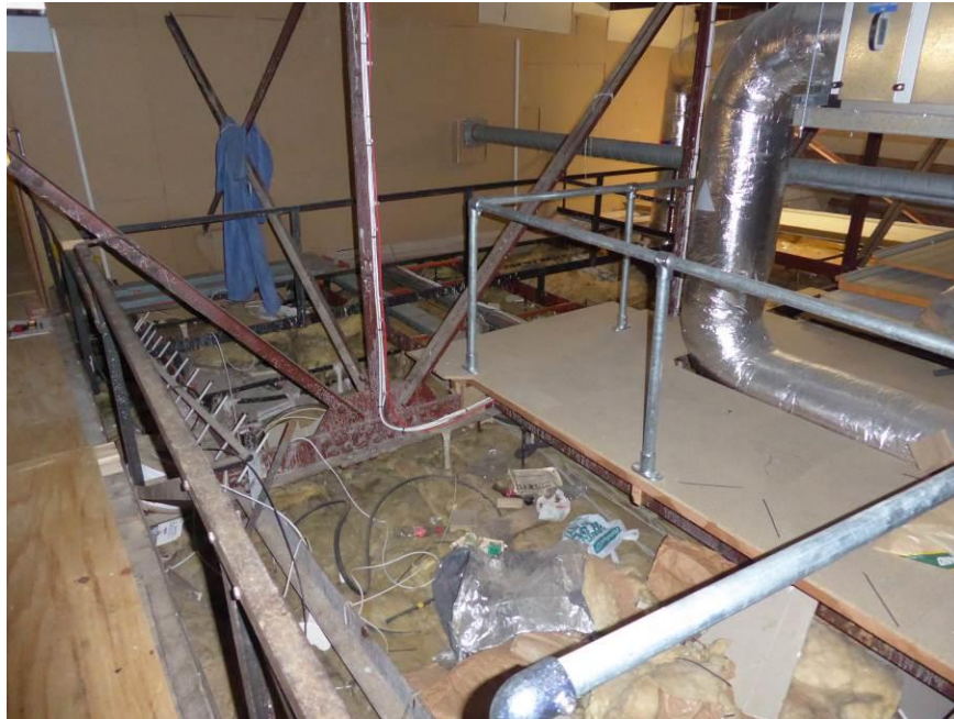
Photo 26 – loft above Alemein Room.
