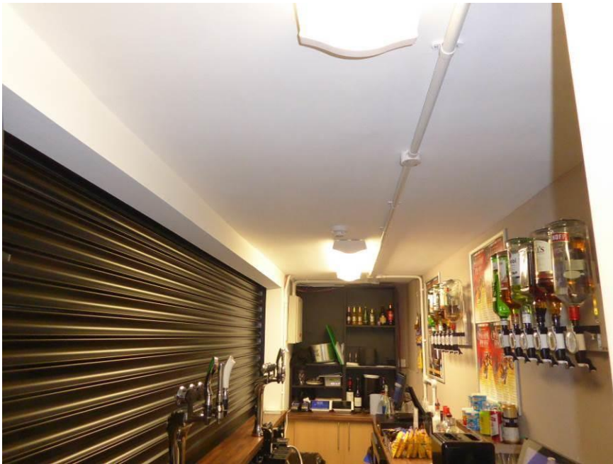
Photograph A10 – Servery ceiling.
