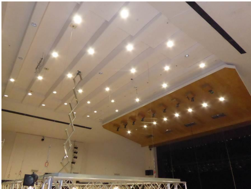
Photograph A12 – auditorium, view towards scene.
