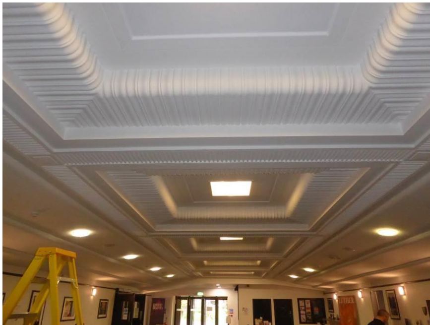
Photograph A8 – Foyer ceiling general view.
