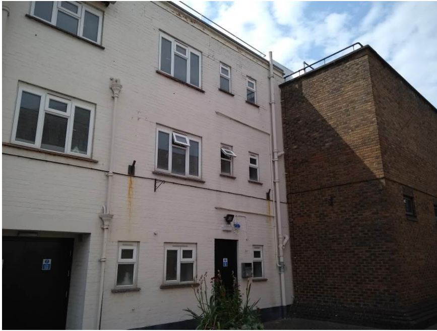
Photograph A3 – East elevation (North end).
