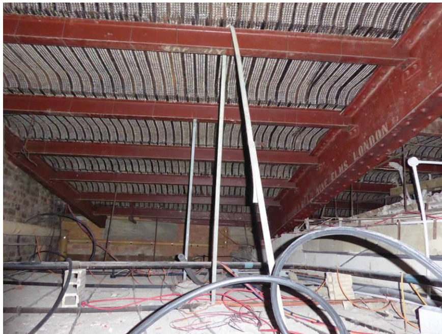
Photo 8 – ceiling void above Kitchen / Servery.
