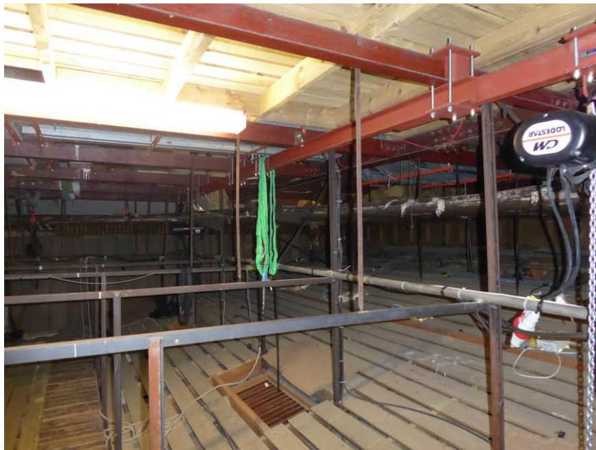
Photo 20 – steel subframe supporting lighting platform.
