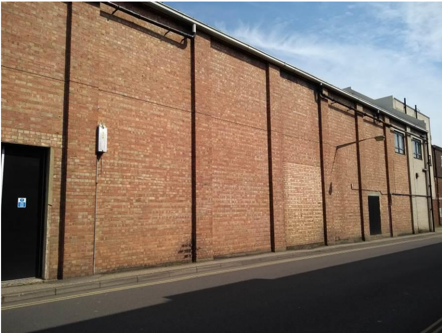
Photograph A6 – West elevation, central part.
