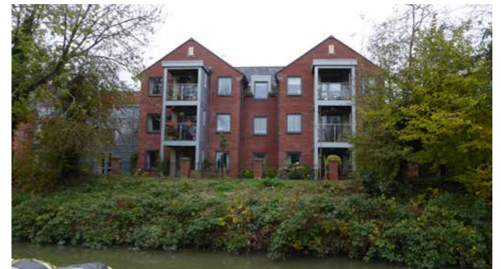
Anstie Court establishes a successful scale response to the canal side and surveillance to key pedestrian routes.
