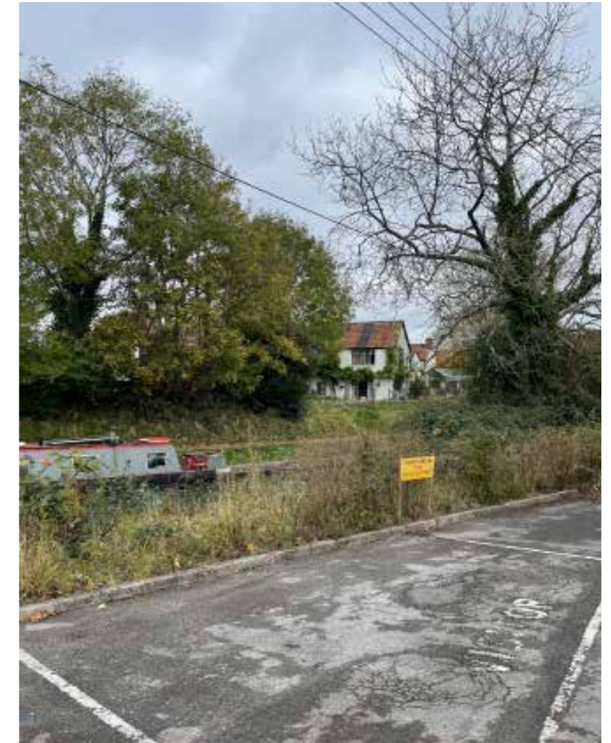
'Stone Wharf' can become an active canal side destination. Existing private car parking spaces would need to be relocated to enable this.
