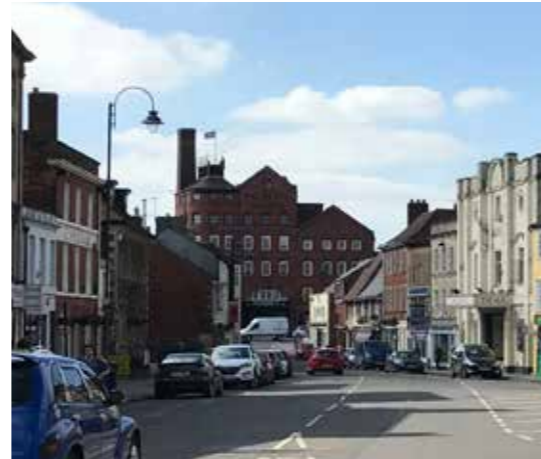
1 Landmark brewery building draws you along Northgate Street
