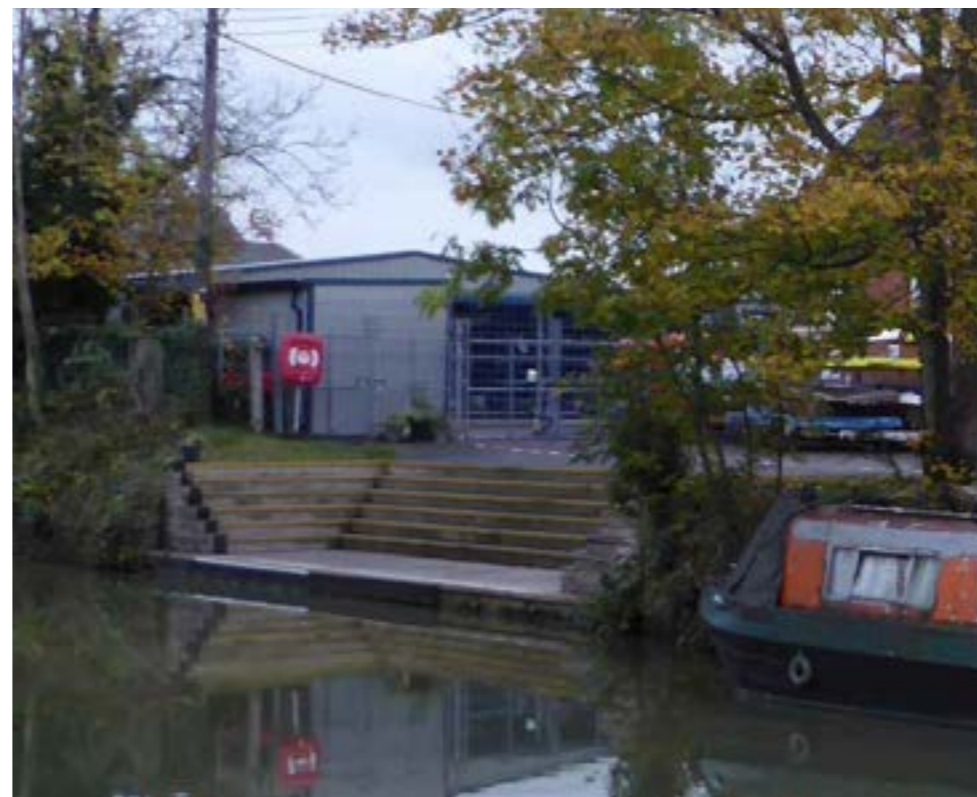
Launching steps provide direct access to the canal, but are currently not wheelchair accessible.
