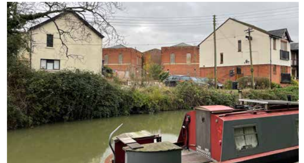
Rear of Assize Court can help improve integration with the canal.
