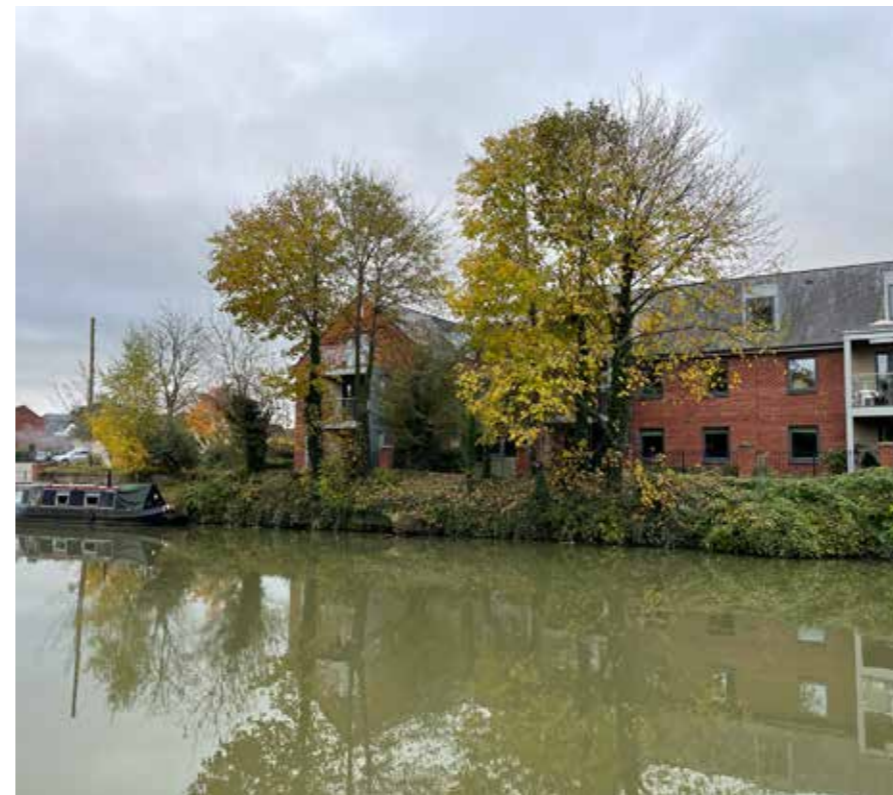
The tranquil and attractive waterside setting of the canal creates a valuable context for new residential uses.
