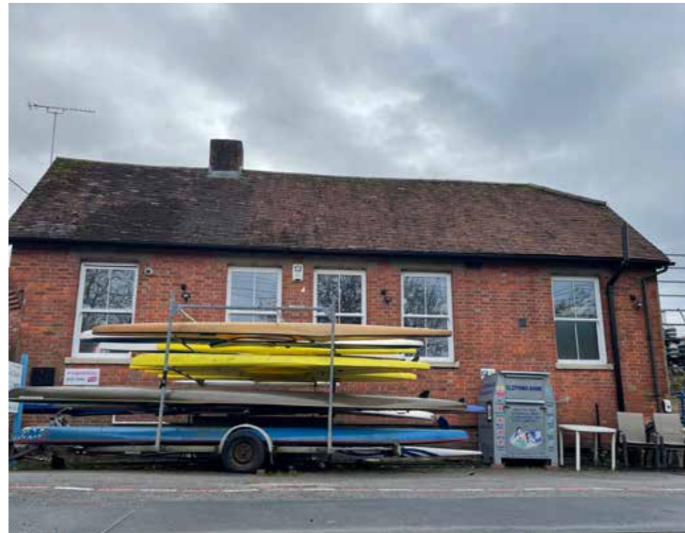
Former road services depot is the hub for 'off water' activities at the club.
