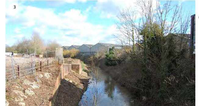
St Stephen's Place / Cradle Bridge
