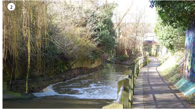
East Wing / Court Street
