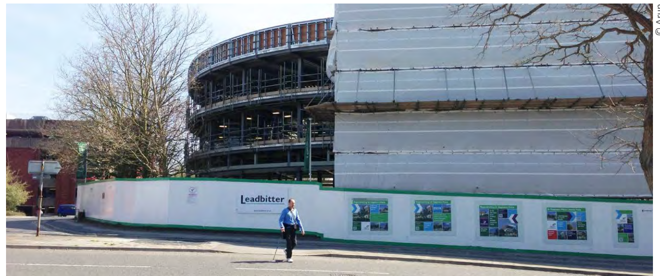
St Stephen's Place - development underway
