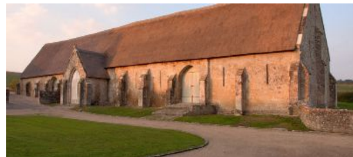
Change of use at the Tithe Barn at Place Farm, before (right) and after (left) renovation from agricultural use to a multi-purpose art gallery and local employment space
