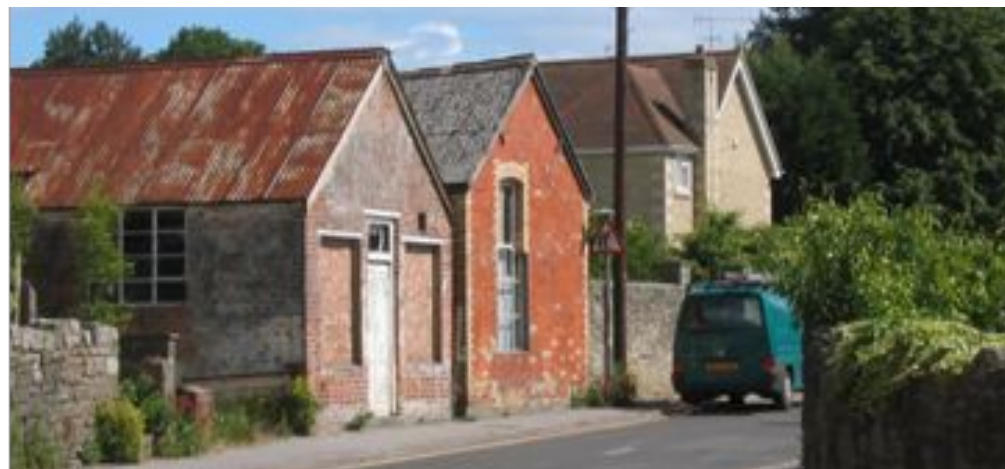
Above: Derelict Overhouse Laundry, 2011
