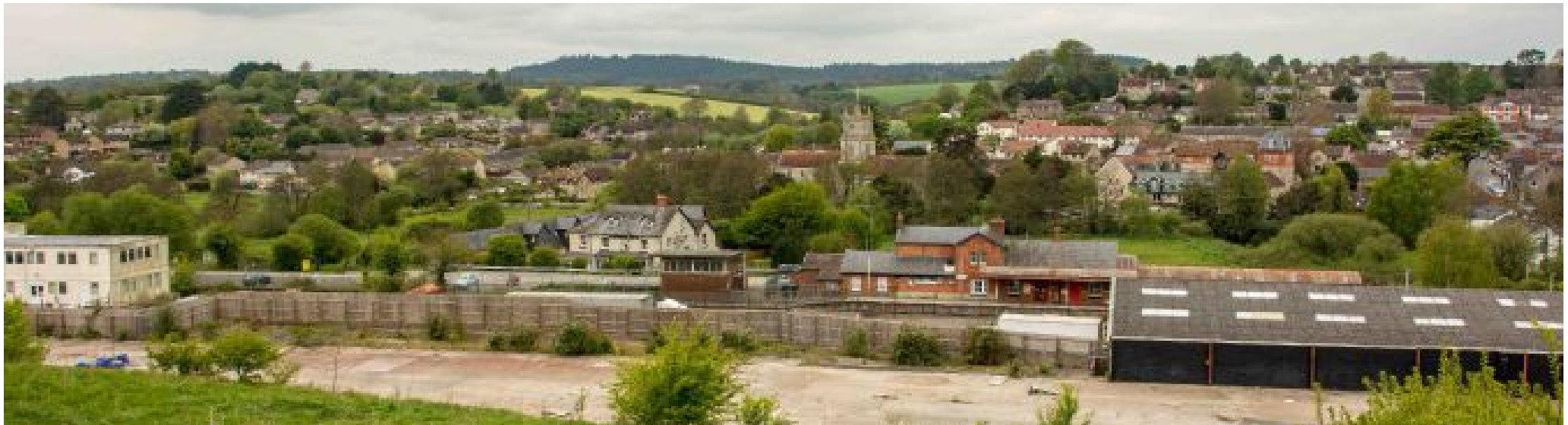
Below: Station Works today, view from the southern side of the railway line
