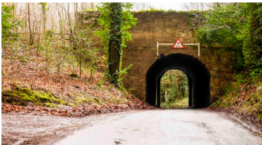
Left: Narrow access from Hindon tunnel on Stops Hill
