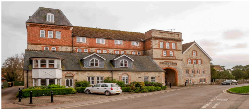
Above: The former Tisbury Brewery, redeveloped as apartments in 1999
