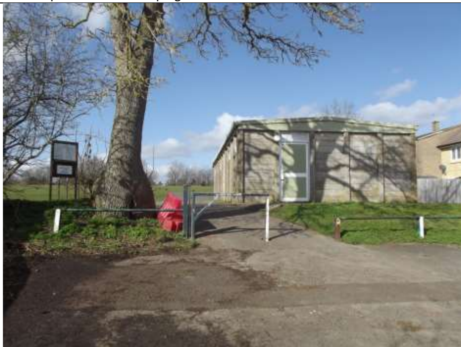
View of northeastern entrance to the Queen Elizabeth Field from Poulton. Poor quality landscape and unattractive changing facility that is remote from the football pitch.
