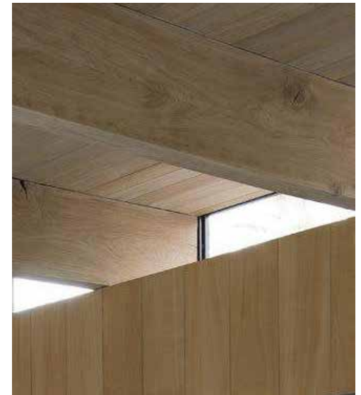
Materials and detailing
