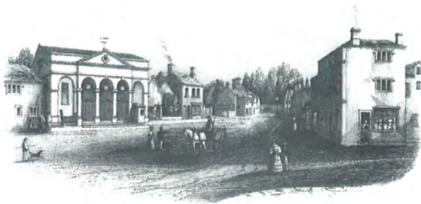
Corsham High Street and the Methuen Market Hall, built in 1783, before its alteration in 1862 to form the present Town Hall.
