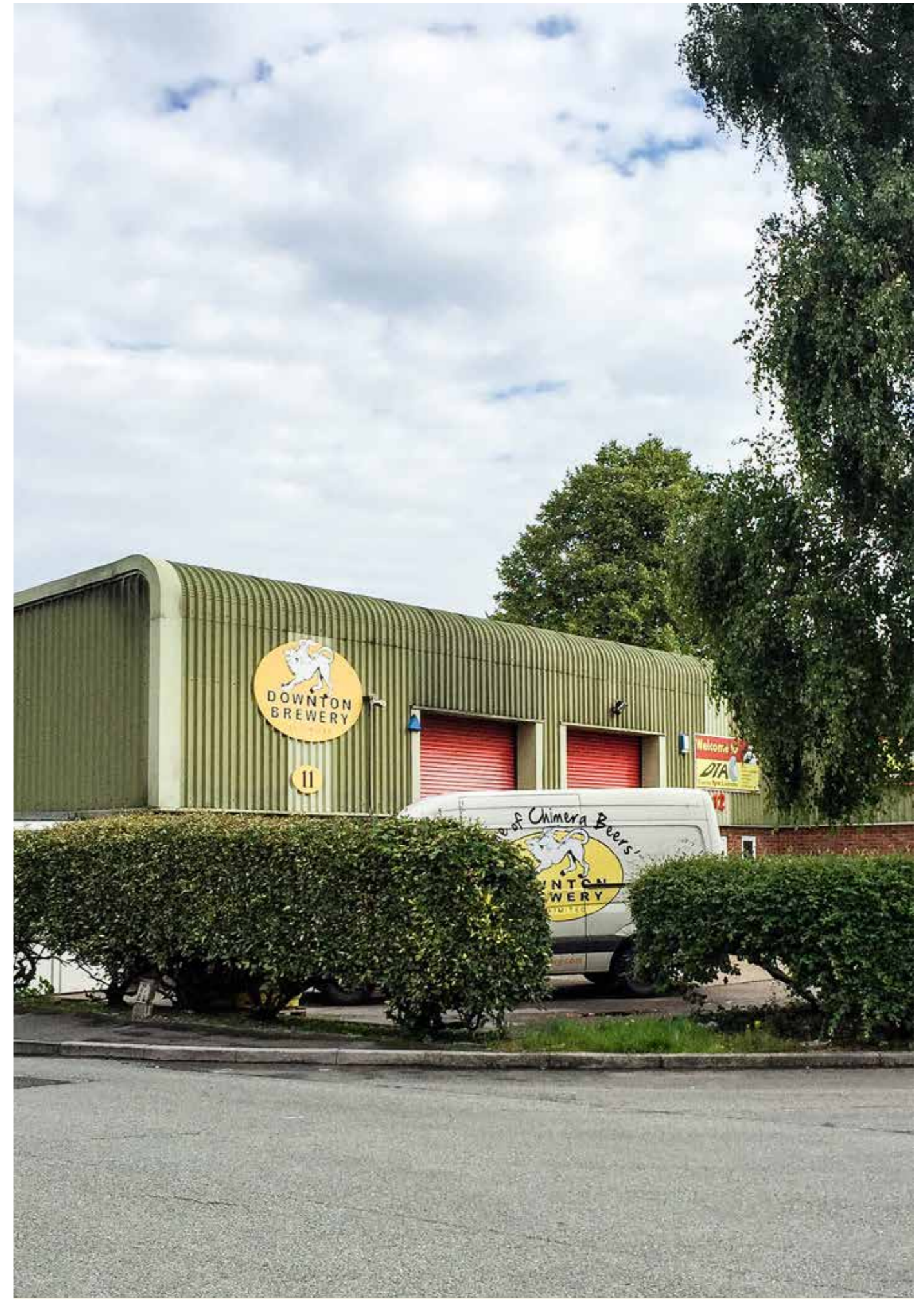
Units at Downton Business Park
