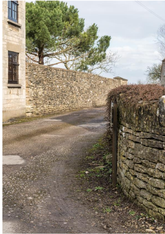
Stone Walls, Coppice Lane
