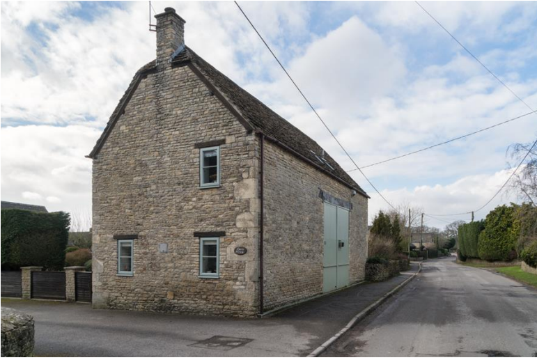
Barn House, South Street
