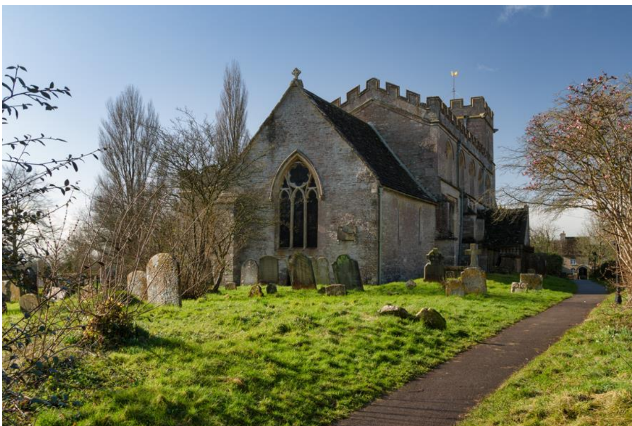
Church and Footpath Looking West
