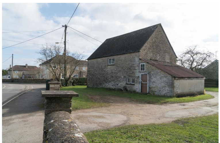
Barn Adjacent to Junction with The Green
