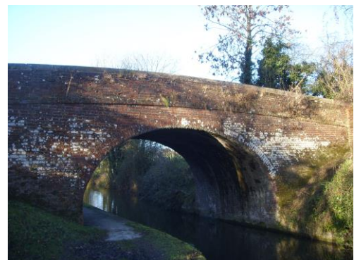
Canal bridges west of the village
