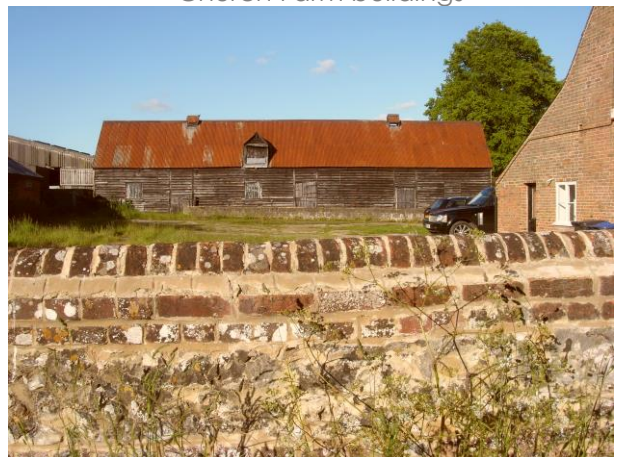
Barn in grounds of Church Farm
