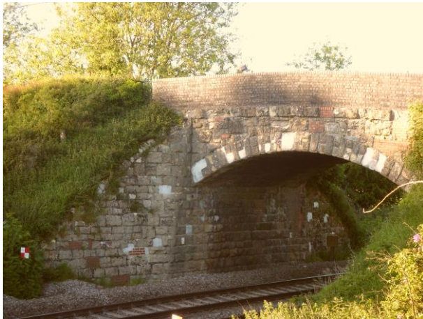
Main railway bridge in village centre
