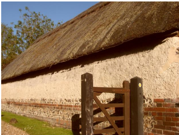
Cob wall of barn at Royal Oak
