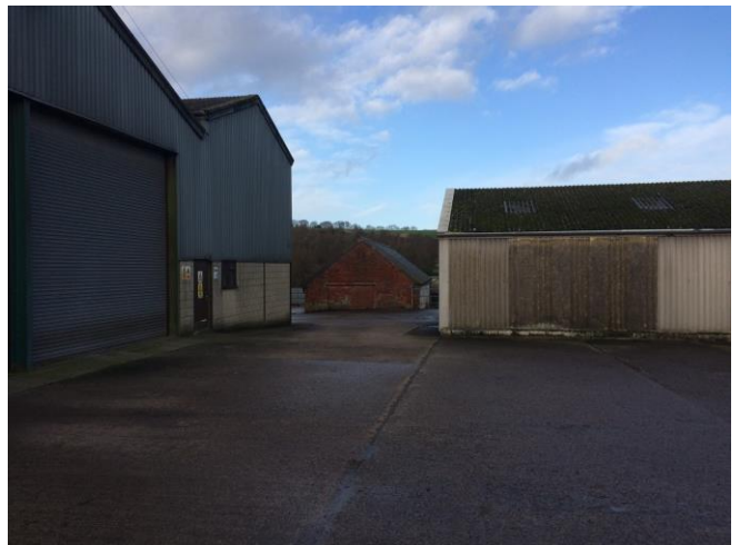
East Wick Farm buildings
