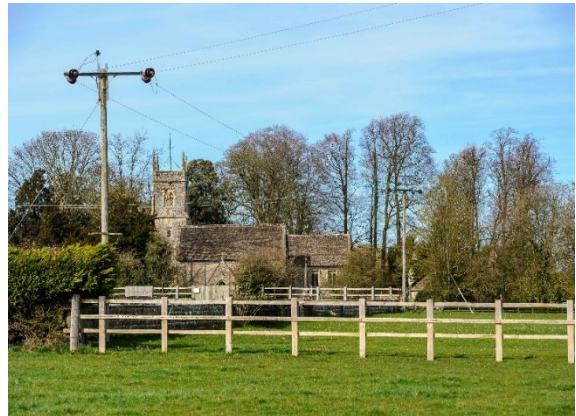
View 10b: From open fields south of All Saints Church, towards the church (close-up)
