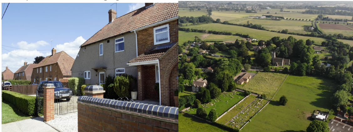
Stone Lane Roofs
