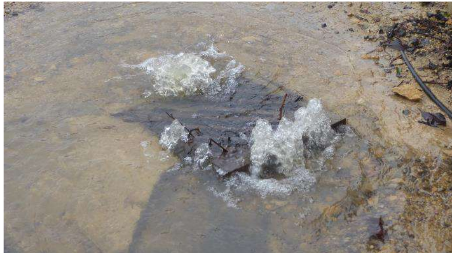
Photo 8: Drainage Overflow, Crudwell
