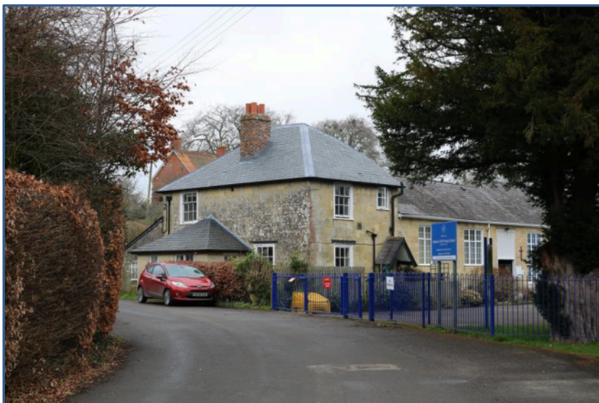
The Old School House and Hindon Primary School
