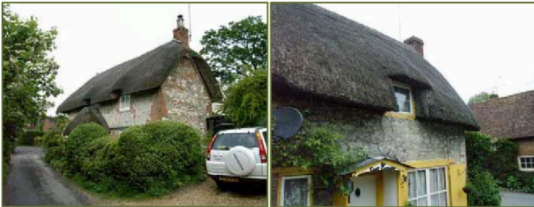
Image 20 (left): Chalk blocks & red brick - Goose Green Cottage and (right): Vernacular chalk build - Cosy Cottage.
