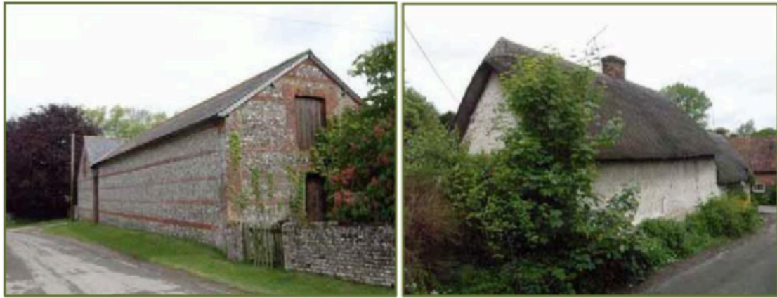
Image 17 (left): Original Brick & Flint at Manor Farm and (right): Cob & Thatch - Cosy Cottage annex, Bulls Lane.
