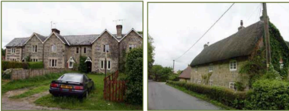
Image 16: 'Reproduction' Brick & Flint in New Town. Figure 22: Green sandstone in South Street.
