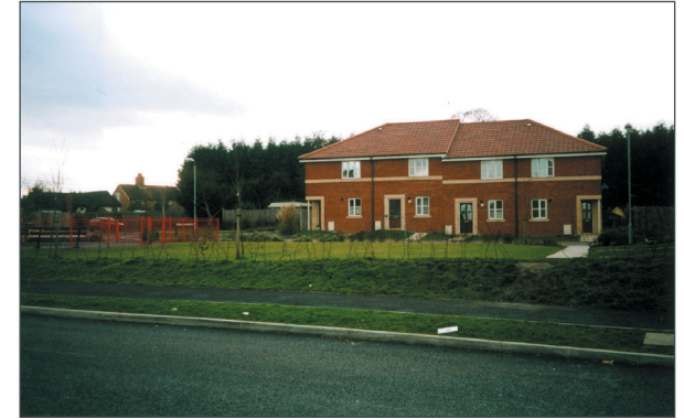
figure 11 Netherleaze, opposite Little Island, is built in contrasting red brick albeit with a similar scale and formal appearance
