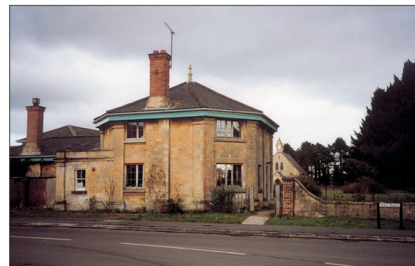
figure 21 The grade II listed Round House stands at the southern end of Vale Road
