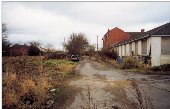
figure 19 The former hospital buildings on the site are derelict and beyond economic repair or reuse
