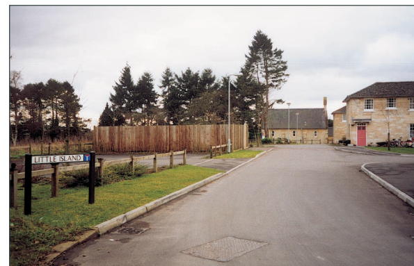
figure 20 The eastern boundary of Little Island comprises parking and clothes drying areas, as well as a toddlers play space, whilst one of the building frontages faces this boundary
