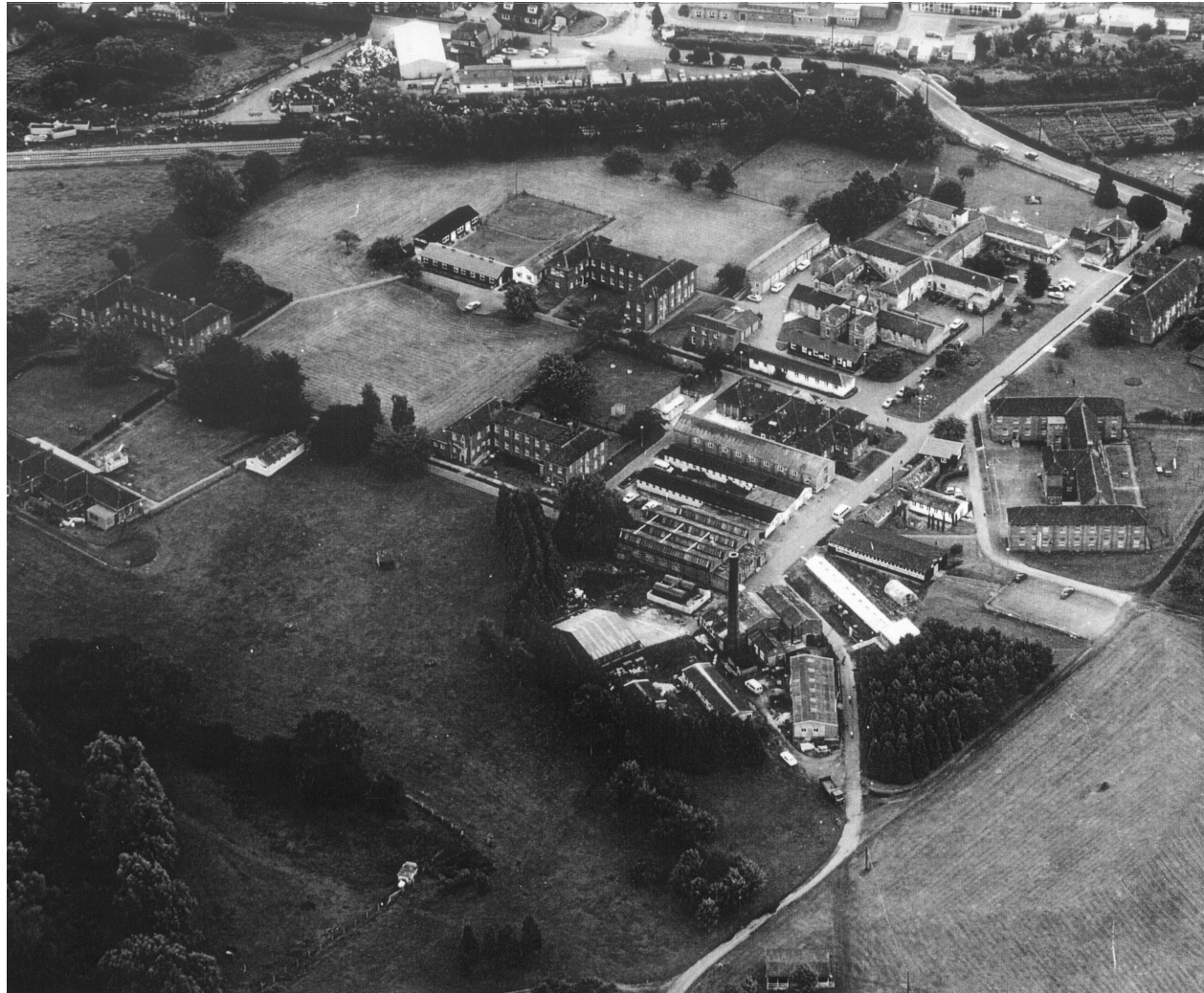
figure 2 The alignment of the access road (now Vale Road), the listed buildings (at Little Island) and most of the mature trees remain from the former hospital
