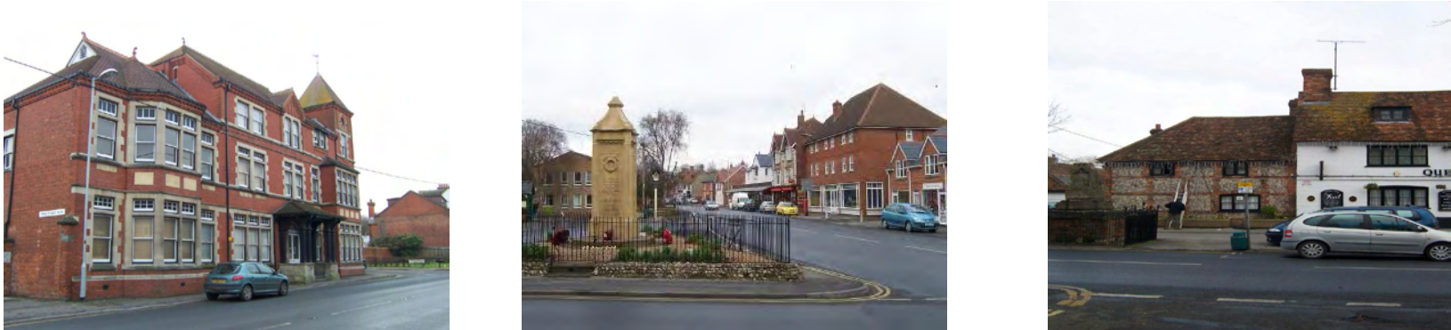
Fig.6. Views around the town centre
