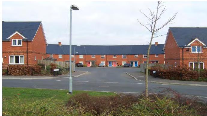
Fig.9. The Sarsen Homes Development to the West of Granby Gardens
