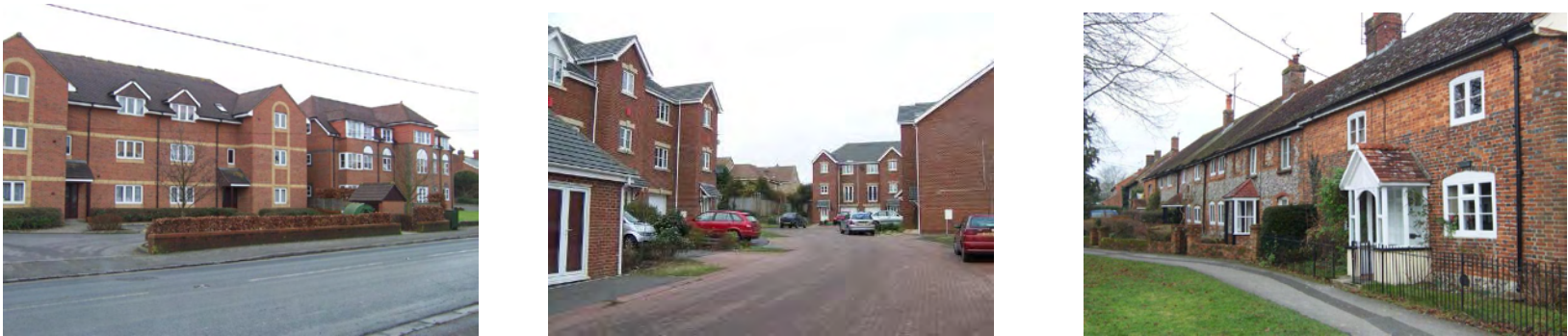
Fig.7. Views of new and old residential development close to the town centre.
