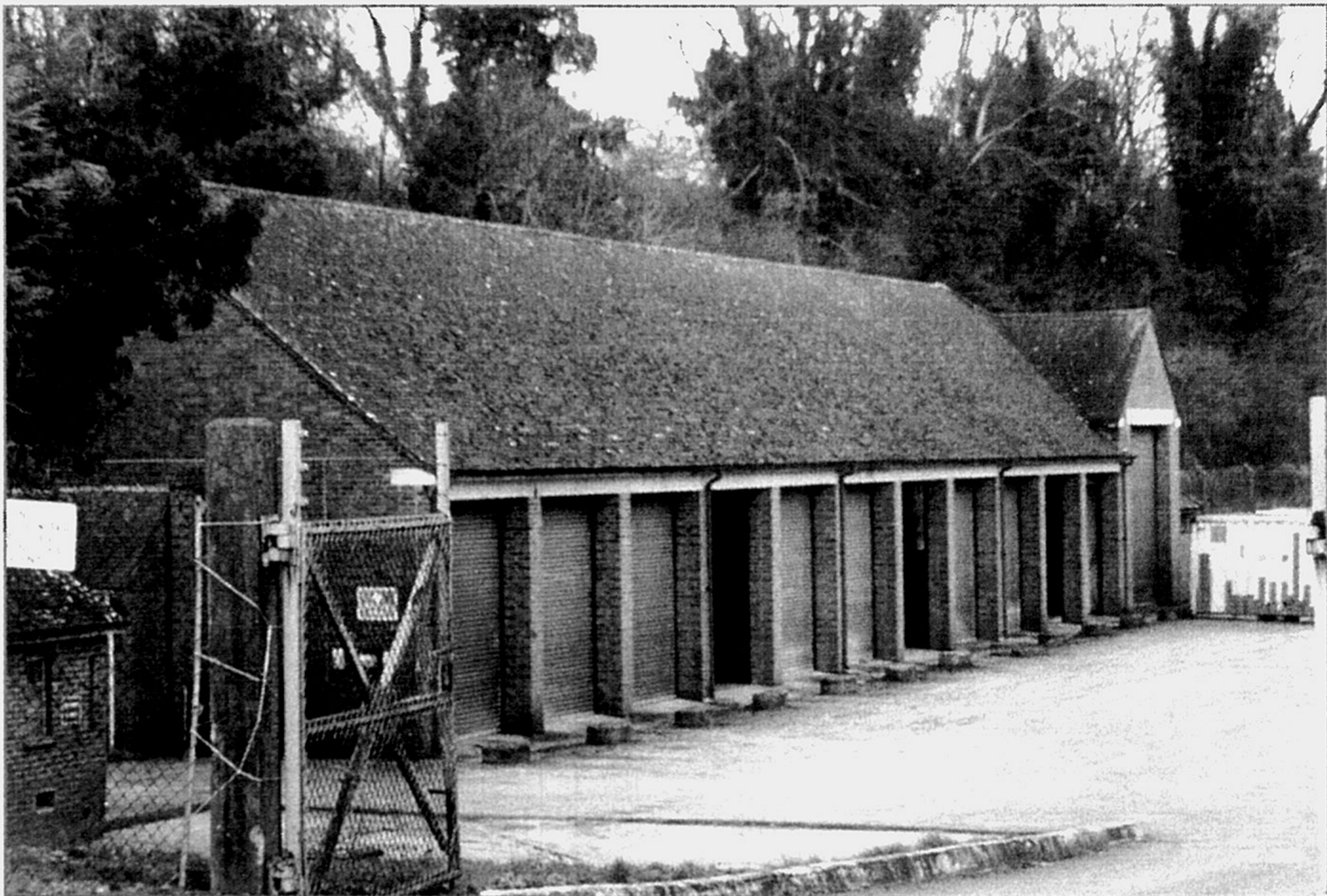
D. Workshops on the MT Yard site, below the HQ North site.
