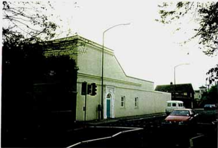
The road frontage of Finch House.
