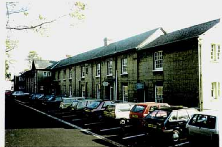
Fonhill - North elevation
