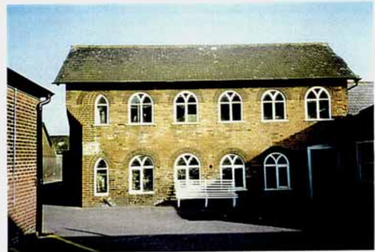
Builders & Painters Store - West elevation
