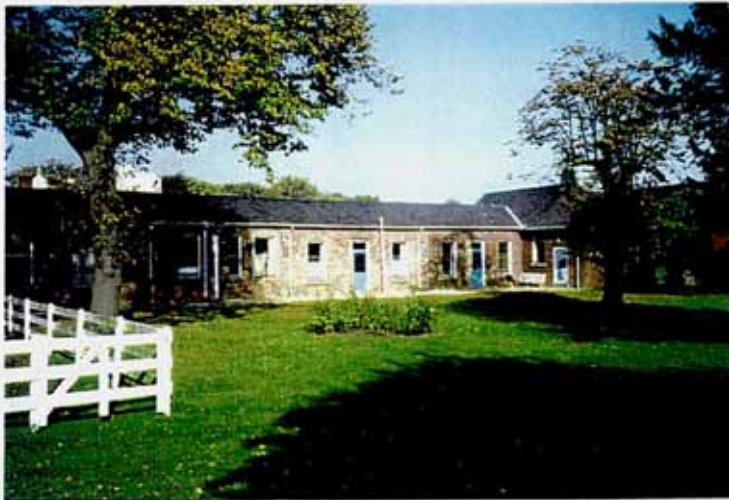
Linford Ward The original building has been much altered
