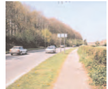
Existing footway on Downton Road
