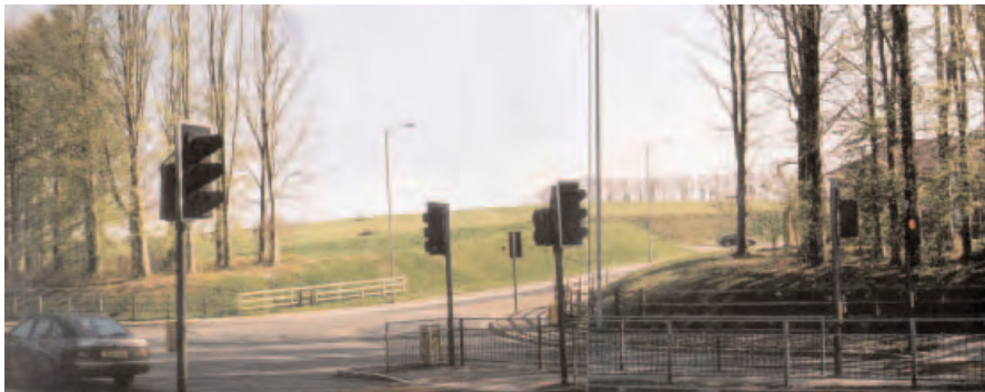
Existing junction of Downton Road and Rowbarrow
