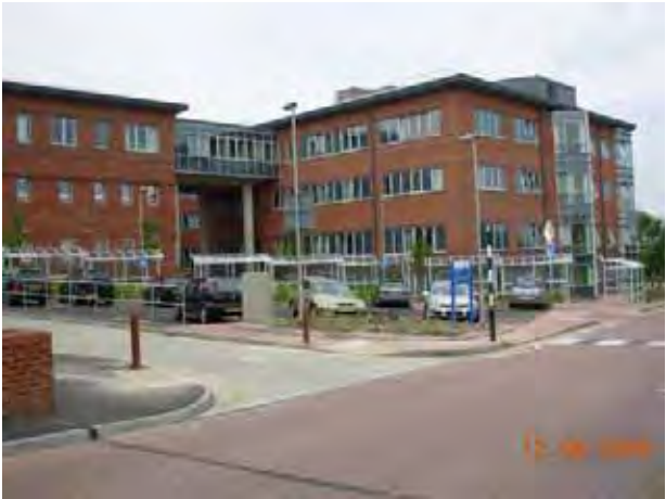
Figure 48 ● New covered walkway
