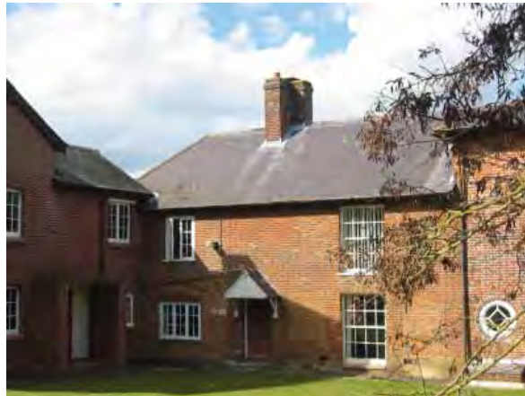
Red House (Side elevation), Durrington
