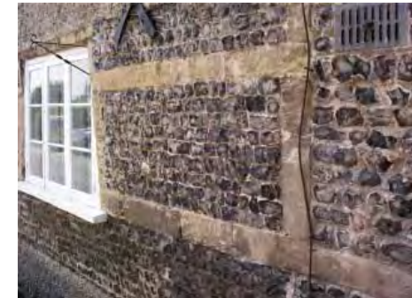
F - High Street, Durrington Relevant design elements: - Flint - Stone banding
