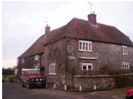
D - Bulford Road, Durrington Relevant design elements: - flint elevations with brick dressings to openings - hipped, tiled roof - prominent central chimneys
