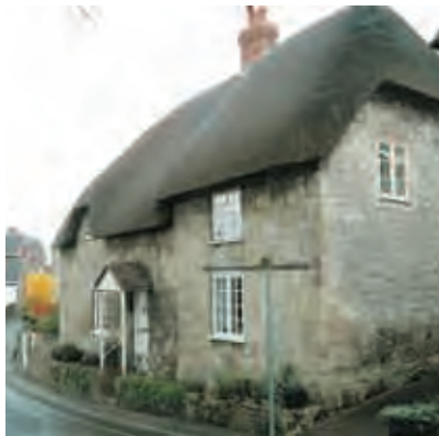
One of the relatively few thatched buildings in Tisbury. Simple cottage in rubble stone with casement windows. Building set back from street with small front garden.
