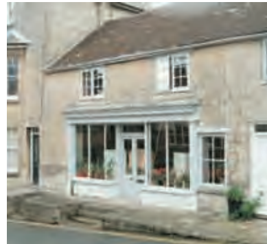
Attractive pressed stone, two storey shop. Adhoc juxtaposition of sash window against shop front adds visual interest.
