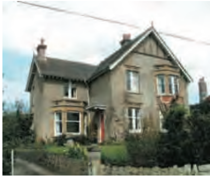
Large detached Victorian villa set within substantial plot. Large front garden gives suburban character. Dressed stone detailing to bay windows and window heads.
