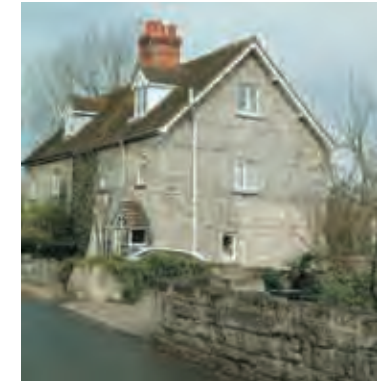
Two and a half storey stone semi detached dwellings set back from road with small garden behind low stone wall.
