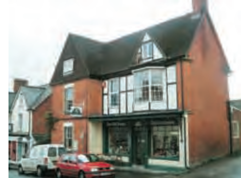
Two and a half storey shop with first floor half timbering detail. Steeply pitched roof with gable features to street with tile hanging.
