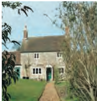
Detached stone cottage with plain clay tile roof. Simple detailing to openings and asymmetrical composition are attractive features.
