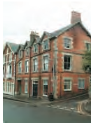
Two and a half storey Victorian town house positioned tight to the back edge of the pavement provides strong enclosure to the street.
