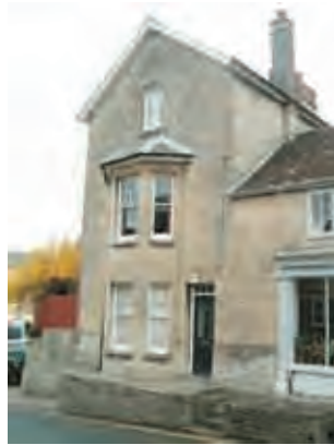
Narrow-fronted well-proportioned two and a half storey Victorian town house gable end to street. Two storey bay provides key feature to elevation in dressed stone.
