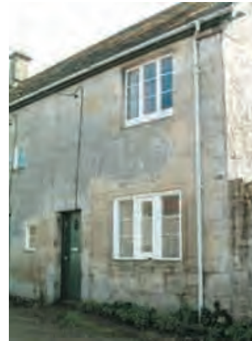
Simple two storey narrow fronted cottage. Simple detailing (originally would have had stone mullioned windows) building tight to pavement edge.
