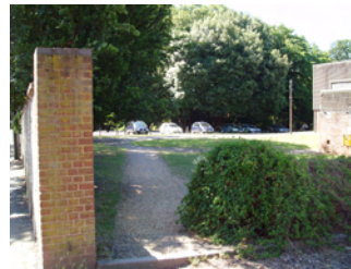
Wyndham Recreation Ground - opening in historic wall
