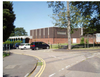
College Street junction
