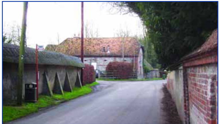
High cob walls such as here with thatch capping, enclose the road and help give a distinct character to the Woodford Valley
