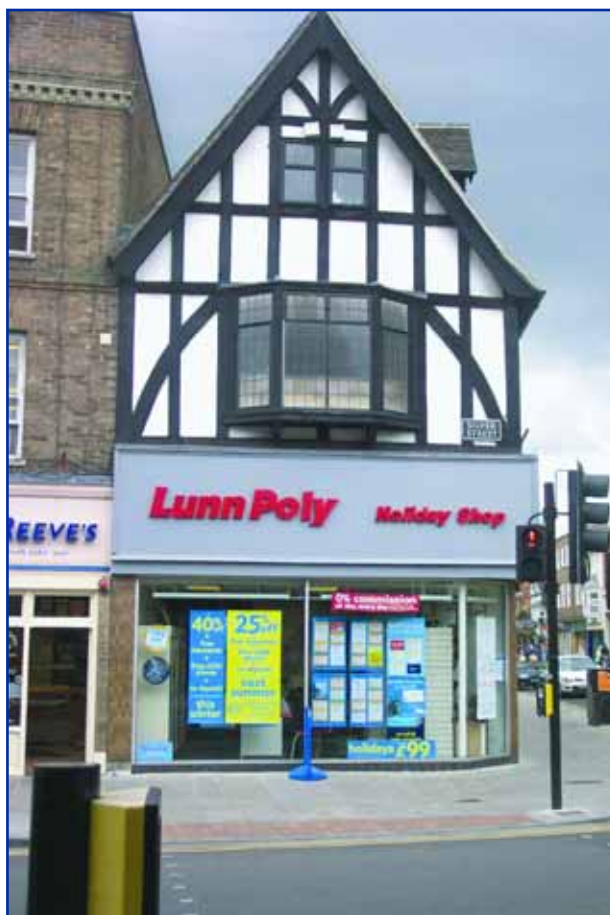
This shopfront fails to respect the building it sits within, it lacks finesse and attention to detail in a manner that detracts from the property itself and the wider setting
