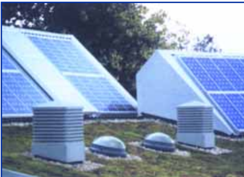
Solar panels and grass roof are used to utilise the sun's energy and provide natural insulation
