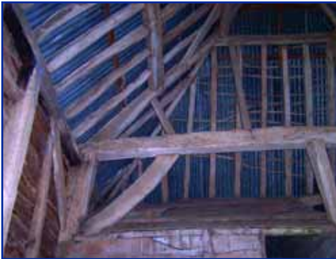
When you live in a listed building all the features both inside and out are protected. Buildings often will have important internal features, such as this timber framed roof structure
