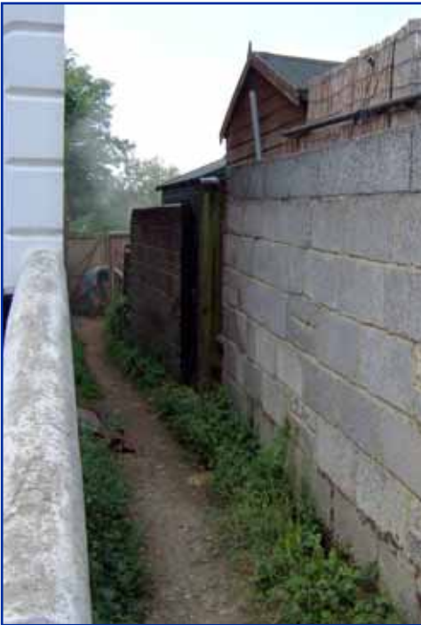
Passages to the rear of properties can provide criminals discreet access into properties and should be designed out from the outset.
