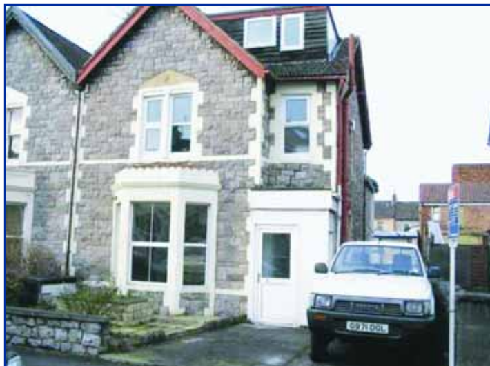
The dormer on this traditional stone Victorian villa is especially crude and ruins the architectural quality of the original fine property
