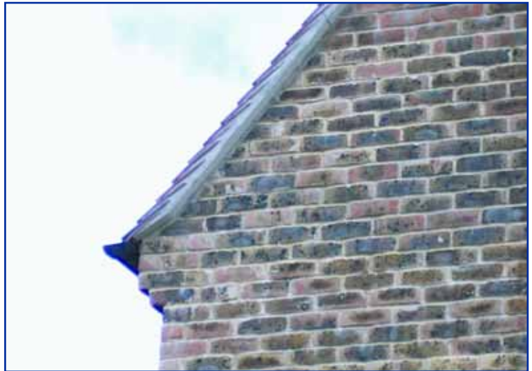
A good verge on a modern house that is narrow not clumsy
