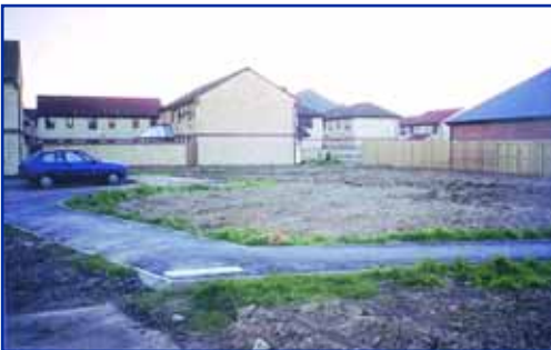
Poorly designed and managed open space
