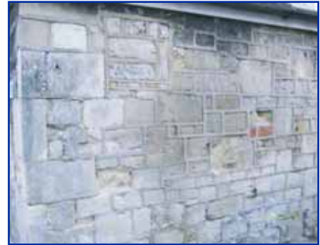
The use of ribbon pointing that stands proud of the stonework is inappropriate, uncharacteristic of the area and spoils an otherwise fine wall
