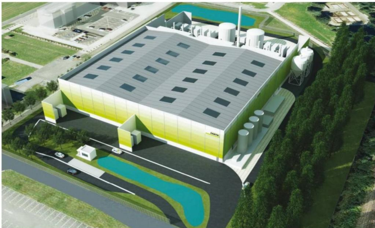
Picture 4.3 Visualisation of proposed energy facility, including pyrolysis units, at Dorset Green Technology Park. Source: New Earth Energy
