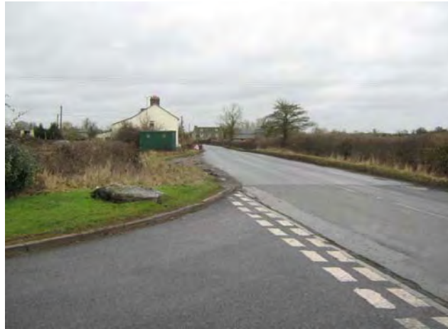
Figure B.1.2.5.2 - Visibility Splay to the North at the Mopes Lane / Cricklade Road Junction
