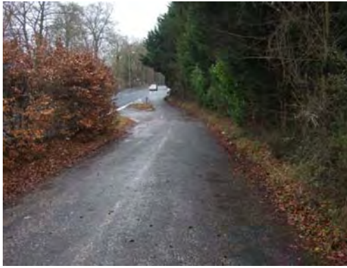
Western on/off slip (view from site)
