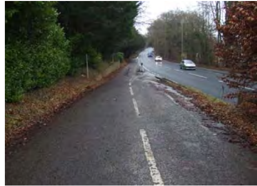
Eastern on/off slip (view from site)
