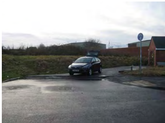
Figure B.2.4.3.3 - Existing Site Access with Electricity Substation
