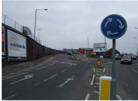
Figure B.5.5.4.3 - Site Access via Mini-Roundabout on Ocotal Way from A4259 Roundabout
