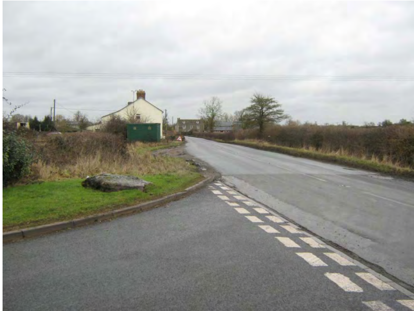
Figure B.1.1.4.1 - Visibility Splay to the North at the Mopes Lane / Cricklade Road Junction
