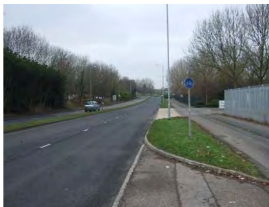
Figure B.5.7.5.2 - View Westwards along Edison Road from the Western Access
