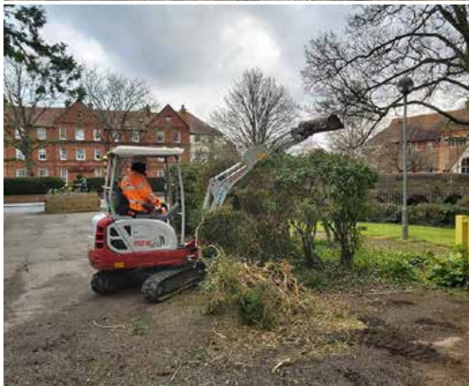
Before and during the clearing of the undergrowth at Crane Lodge
