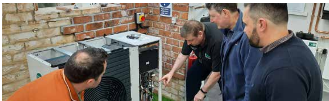
Council surveyors learning about the benefits of heat pump technology
