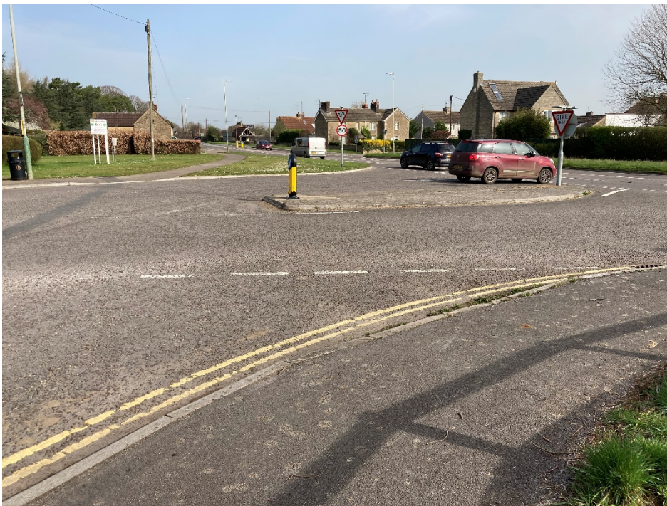
Figure 2-17 – A429 Church Lane junction
