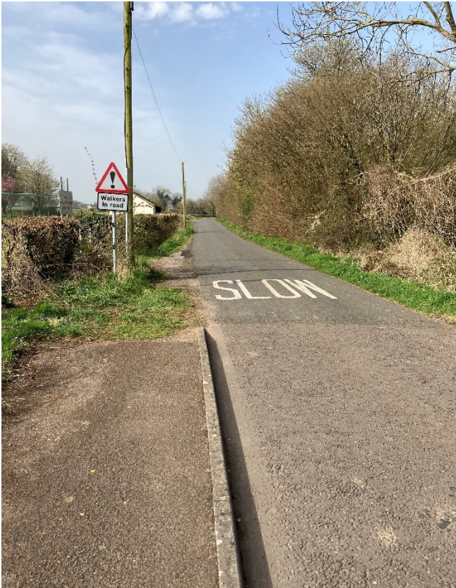
Figure 2-18 – End of footway on Church Lane towards Stanton St Quintin
