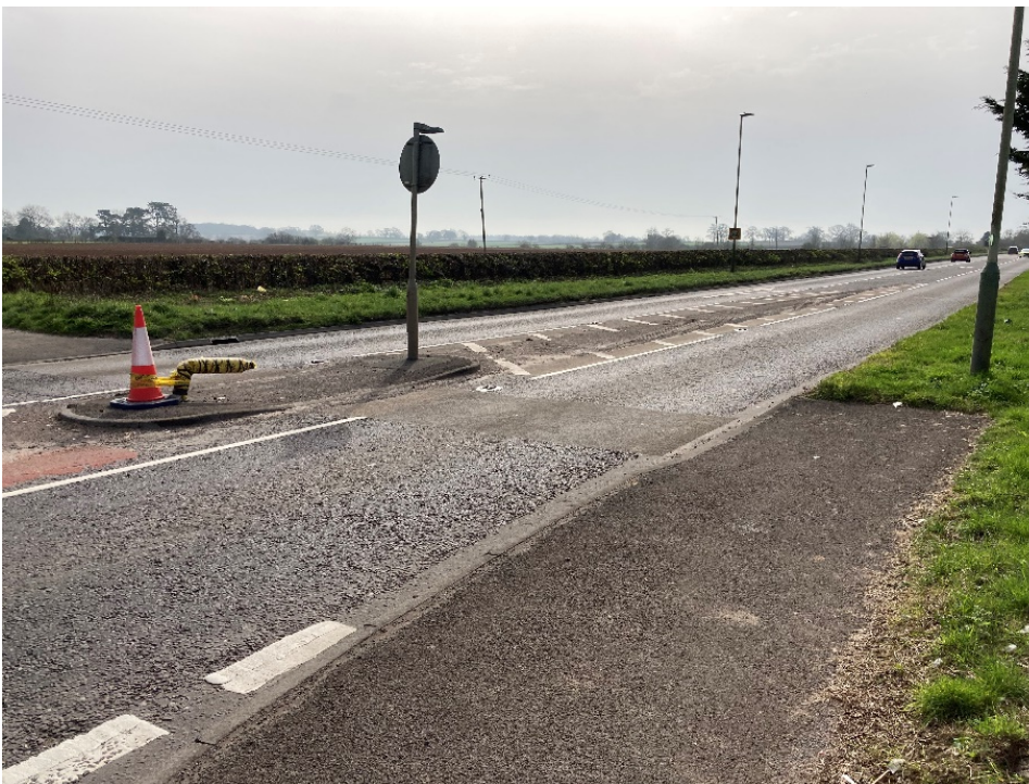
Figure 2-15 – A429 uncontrolled pedestrian crossing south of Church Lane
