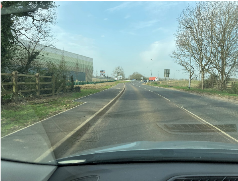
Figure 2-12 – New footway on B4122 between Chippenham Pit Stop Services and Chippenham Gateway development
