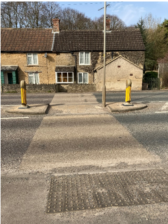
Figure 2-13 – A429 uncontrolled pedestrian crossing north of Seagry Road
